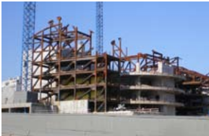
The Kauffman Center for the Performing Arts Center under construction
