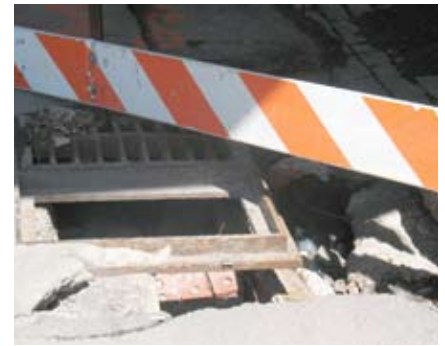
Broken catch basin in the West Bottoms
