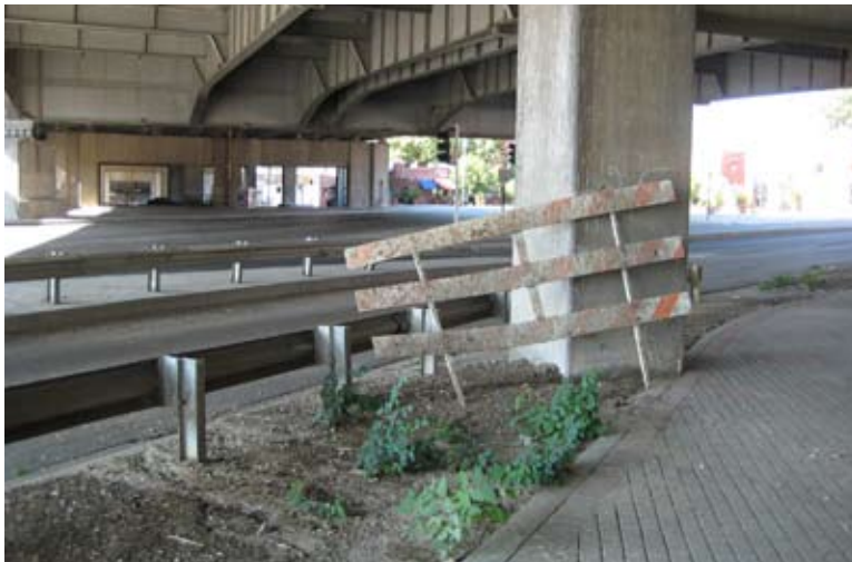
Dirt, debris and broken glass litter the sidewalk and add to the perception of an unsafe environment in this underpass.
