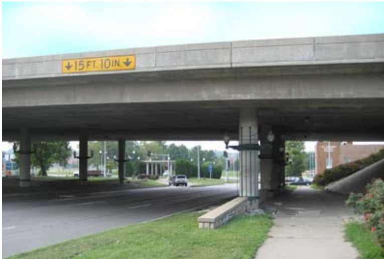
Well-defined sidewalks and lighting help mitigate the barrier between the Paseo West and 18th and Vine neighborhoods.
